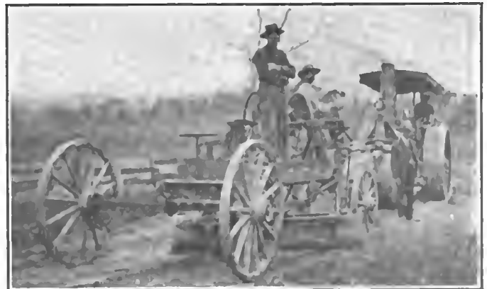
Fig. 4—Equipment for road-building caught in the act
